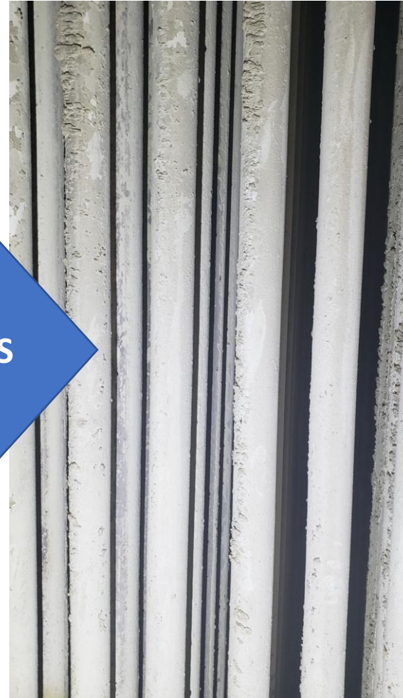
After 7 weeks Vortex cleaning: - ash hopper plugging eliminated - superheater ash deposits eliminated - outperformed (6) sootblowers
