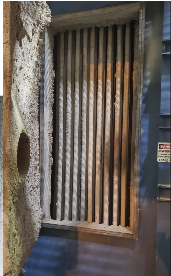
After 7 weeks Vortex cleaning: - ash hopper plugging eliminated - superheater ash deposits eliminated - outperformed (6) sootblowers
